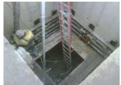
normal excavation, the inside face of the sheet pile walls would have to be a couple of feet from the outside face of the concrete walls. The space is needed for the bracing system and for formwork. LD Docsa wanted to eliminate the bracing system and use the sheet piles and the concrete walls together in a unique configuration. The steel sheet piles were used
